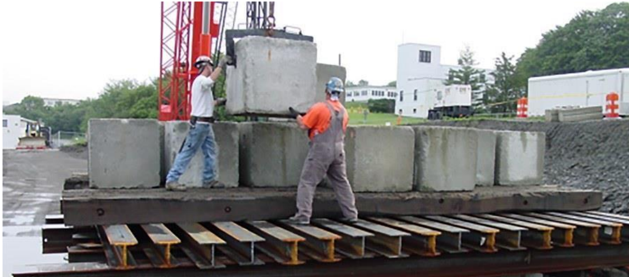
Layers of concrete blocks supported by H-Beam (no. and sizes varies according to required load)
